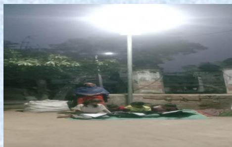
Installation of solar light through project support
