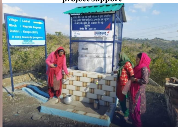
Installation of community water tank through project support
